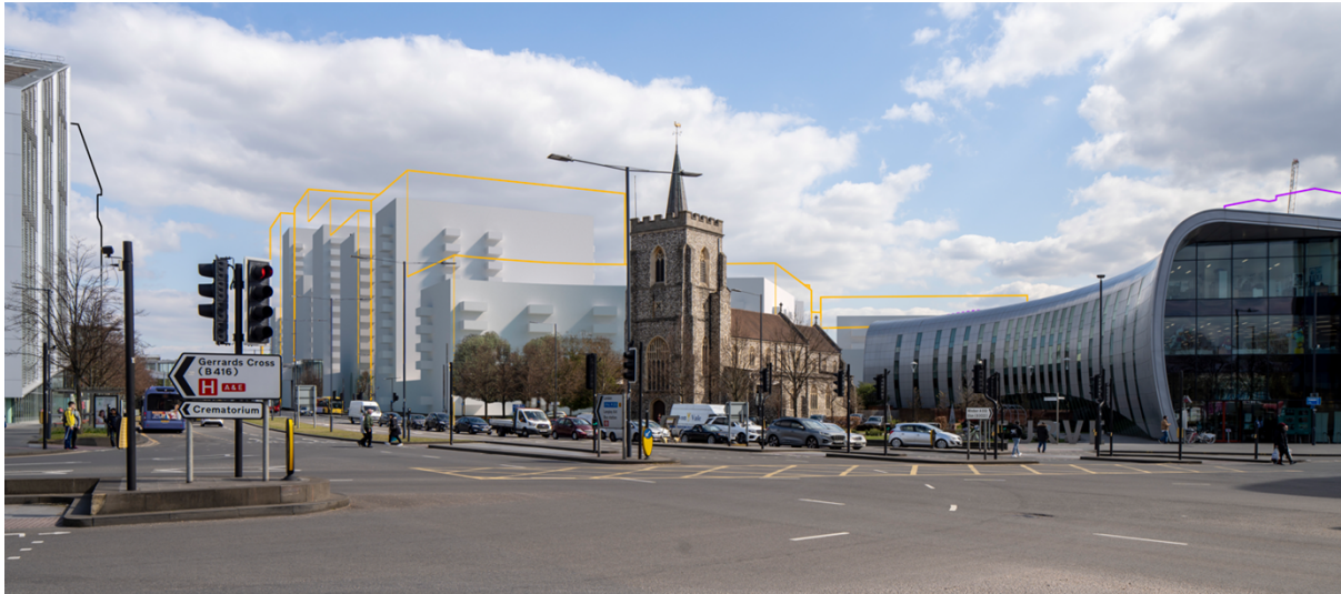
Fig 38: TVIA view of Grade II Listed St Ethelbert's (with development in background)
